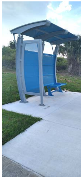
Installed covered bus shelters with raised elevation (GAT 9)
