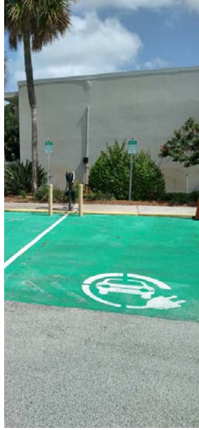
Installed 3 EV charging stations (GAT 4)
